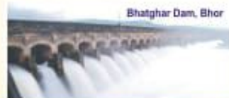
Bhatghar Dam, Bhor
